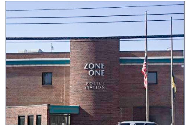
Zone 1 Police Station, Brighton Road.
